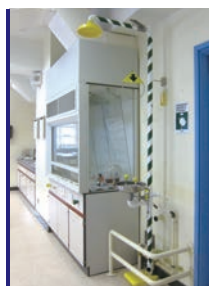
Emergency Shower and Eyewash Biology Lab, Physics Lab and Chemistry Lab
